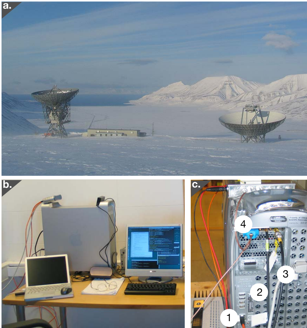
Figure 14.: The space debris receiver at the EISCAT Svalbard radar. Panel (a) shows the 32 m fully steerable antenna (left), the site building, and the 42 m magnetic field aligned antenna (right), at the altitude of 420 m on a north-facing slope of the Breinosa mountain, at latitude 78.153^{\circ}\text{N} . Panel (b) shows the Macintosh G5 analysis computer, the console screen and firewire disks in the site's control room. Panel (c) shows the Macintosh G4 measurement computer, with the external connections: gigabit ethernet to the analysis computer (1), IF2 signal from the radar's analog receiver (2), phase-locked 10 MHz frequency reference signal from the radar's frequency distribution system (3), and the receiver protector bit from the transmitter radar controller (4).
